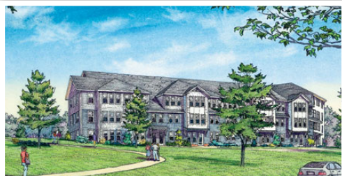
Residences at Canal Bluffs, Bourne
