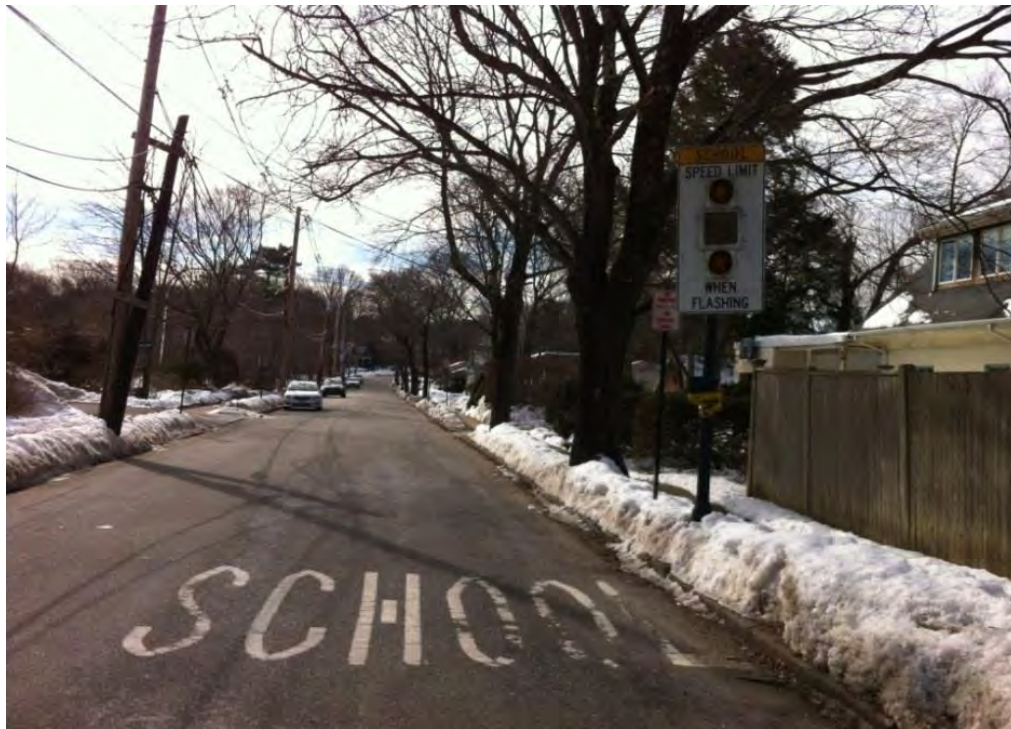
Looking south on Beethoven Avenue. Flashing beacon is non-operational and may cause confusion due to the one-way northbound operation during peak school periods.
