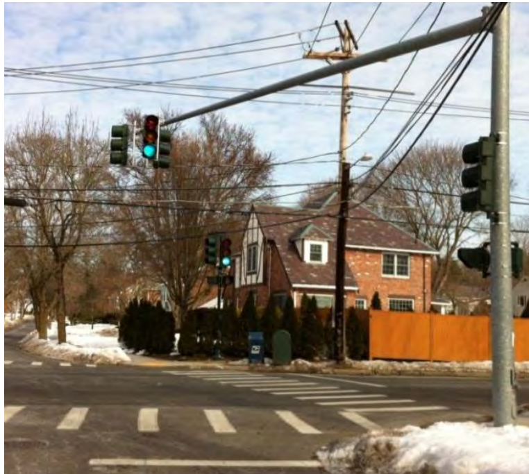
Traffic signal heads have no backplates, which would enhance signal visibility
