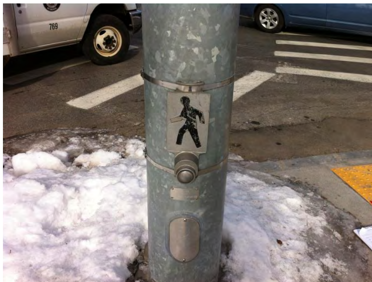
Pedestrian push-button and signage is non-compliant with the latest MUTCD and ADA standards
