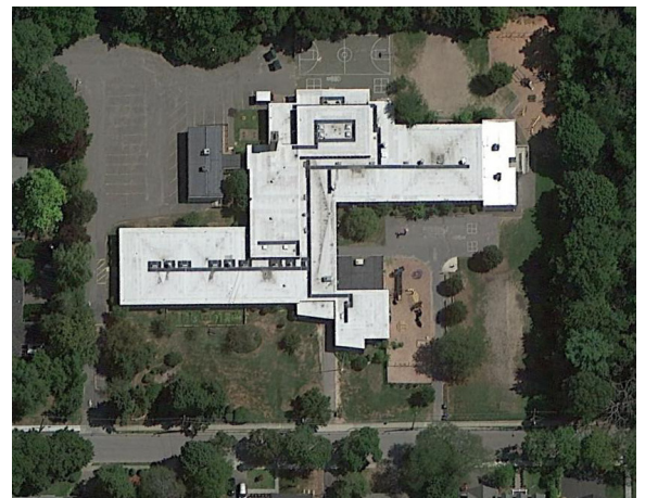
Aerial View of Existing Zervas ES
