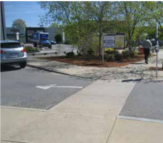
Continuous sidewalk across a driveway
