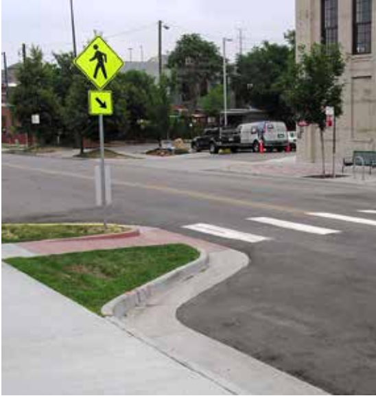
Curb extension at a mid-block crossing
