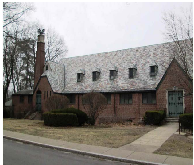
View of existing Church from Short Street
