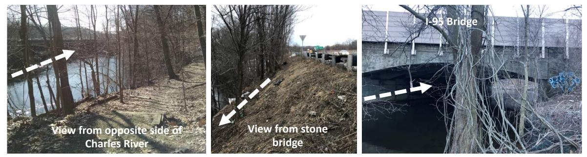
Bringing trail under I-95 bridge would require a cantilevered boardwalk. Challenges: vertical clearance, permitting, lighting, comfort
