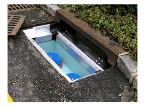
Installed 32 Catch Basin inserts to remove pollutants from stormwater discharge into Crystal Lake.
